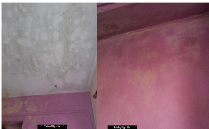
[Table/Fig-3a,b]: Damp roof and walls showing fungal growth
